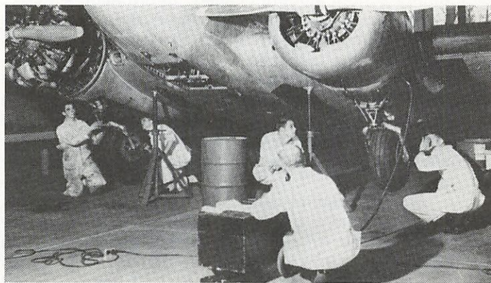
Performing a landing gear retraction test. Left to right: Clayton Holteen, James Longacre, Lewis Mortensen, Mel Gaskill, Darrel Mansveld.
