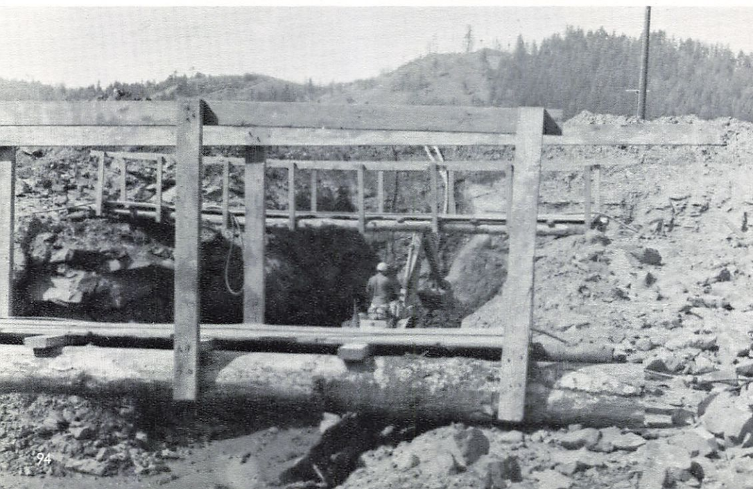
Looking down into one of the many tunnels that will connect all the buildings on the new campus.
