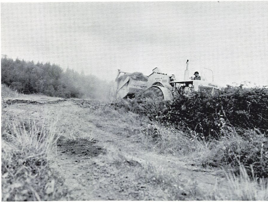
The first grading of the new campus site. Photo taken last year.
