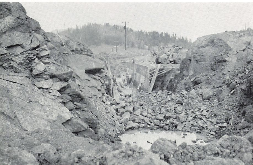
Scene after blasting way for a tunnel in the rocky field.
