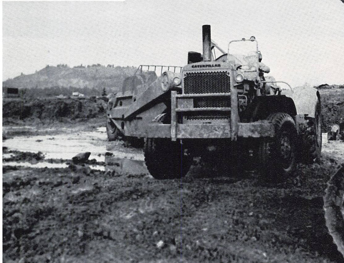
Heavy equipment clears the way for the new buildings.
