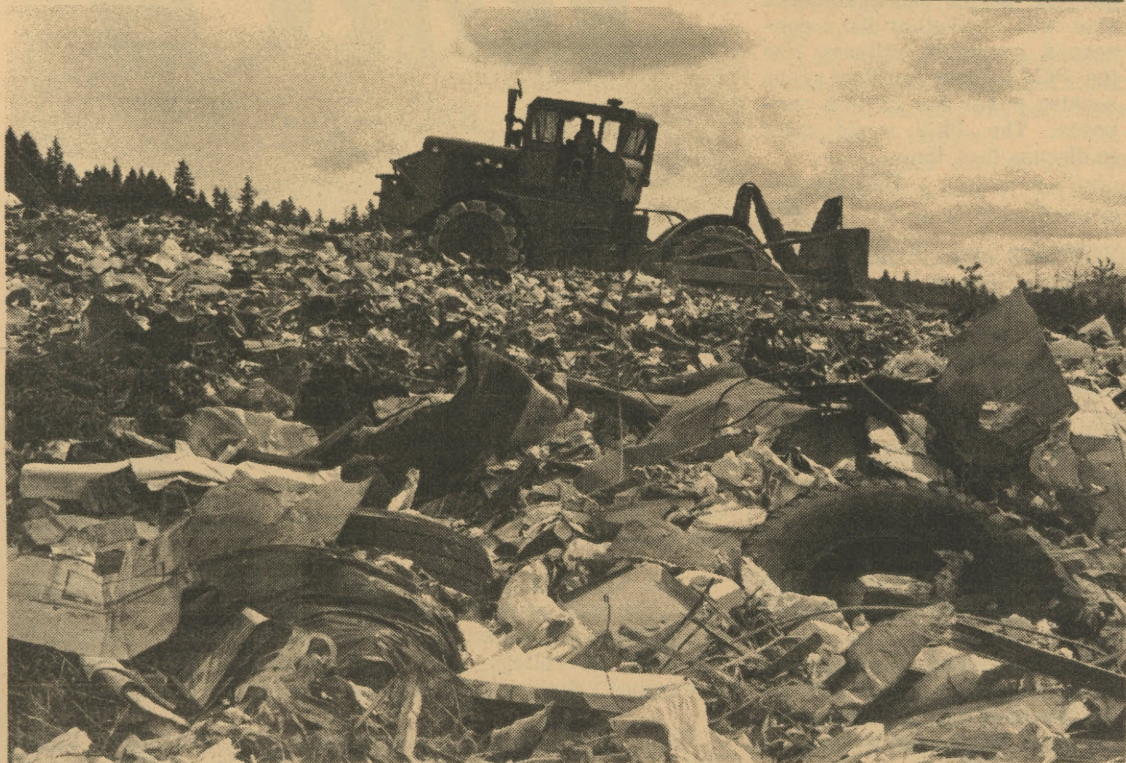
BULLDOZER PACKS THE GARBAGE at the Lane County Dump (Day Island "Sanitary" Land Fill).
