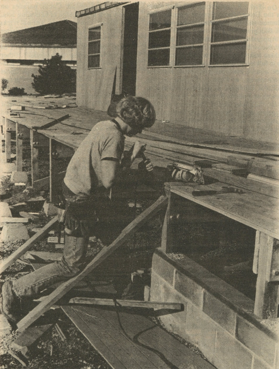
Wes Norbo adjusts the bracing holding the deck.
