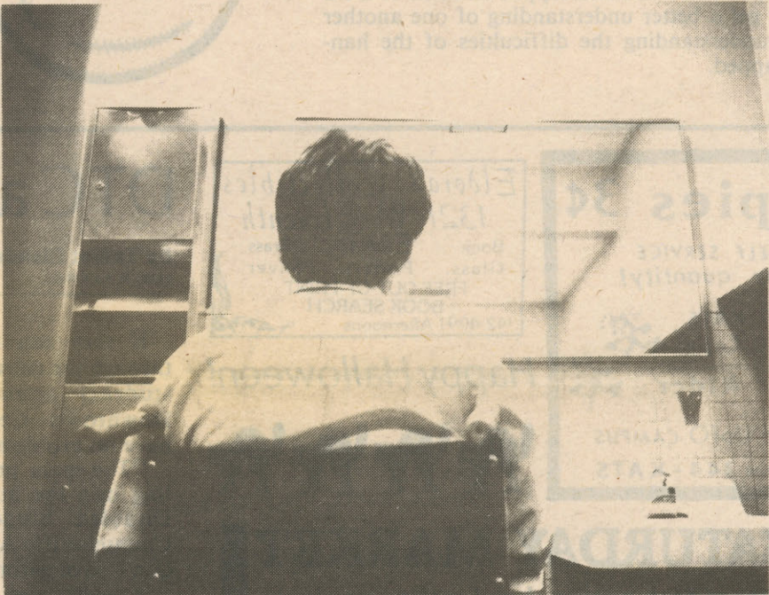
Restrooms: Sinks are placed to far back to reach, mirrors are too high to see in, and stalls are not wide enough to maneuver wheelchairs in easily.
