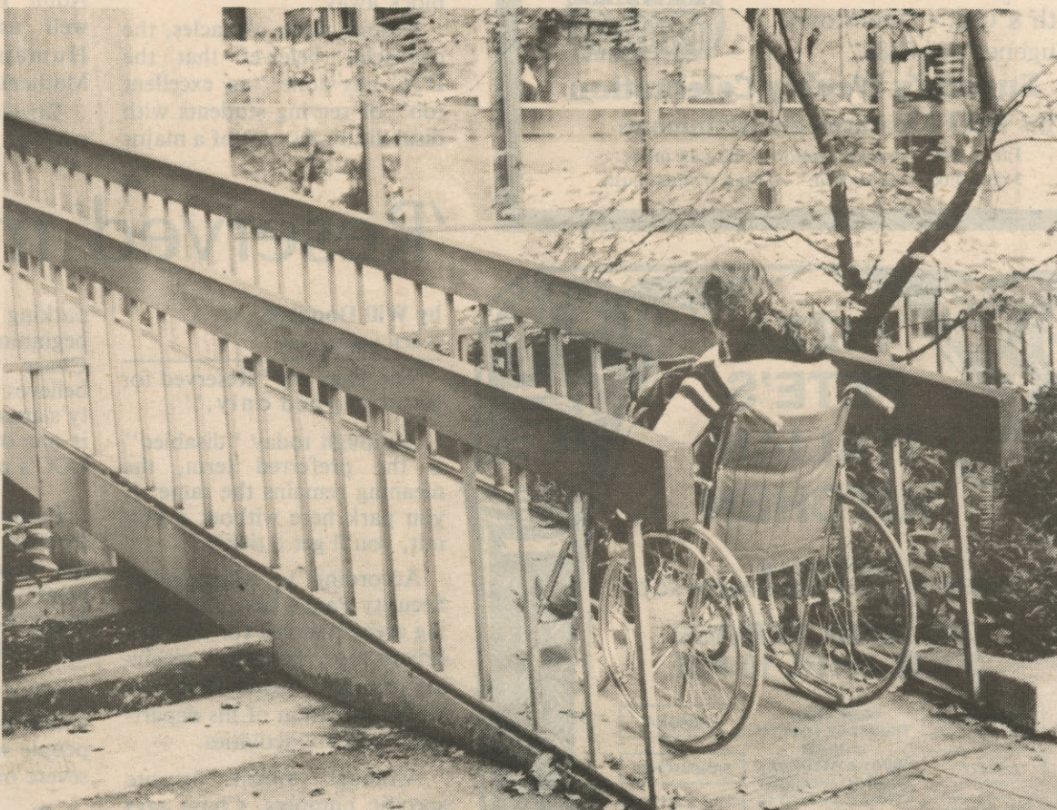
Ramp into KLCC: Built over the maximum one inch per one foot grade, the ramp is difficult to traverse.
