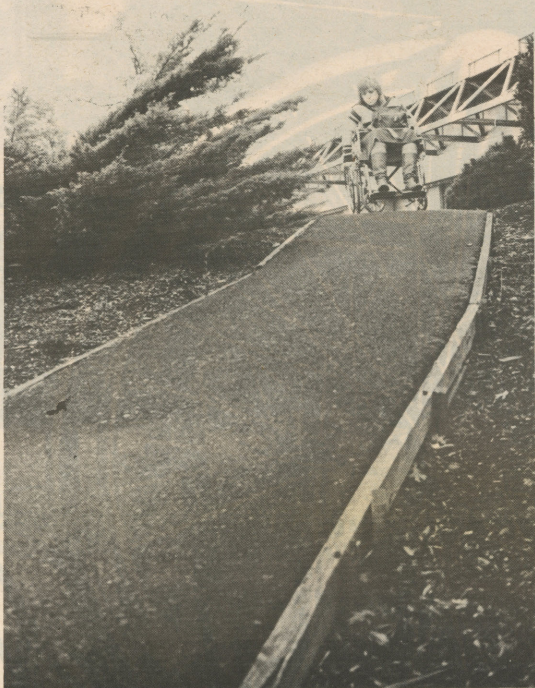
Access ramp behind Performing Arts Building: Steep slope makes it unsafe for wheelchairs.
