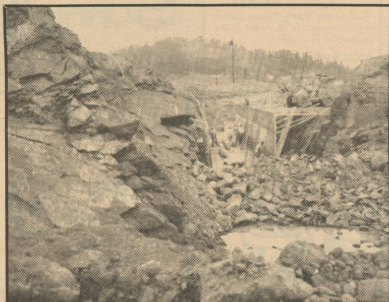
The first stage of construction involved the excavation of nearly one mile of service tunnels under the buildings. The work was not visible from 30th Avenue for several months.
