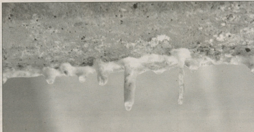
These "soda straws," located outside LCC's cafeteria beneath its upper deck, are so named because of the narrow and hollow core. The cause is water seeping through the upper deck and as it vaporizes leaves behind the minerals that form the stalactites. Photo by JB BOTWINICK/The Torch
